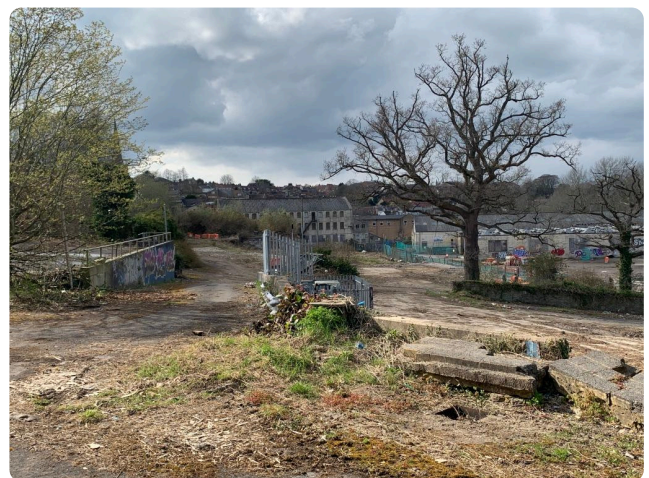
Current Saxonvale site – Credit: Mayday Saxonvale
