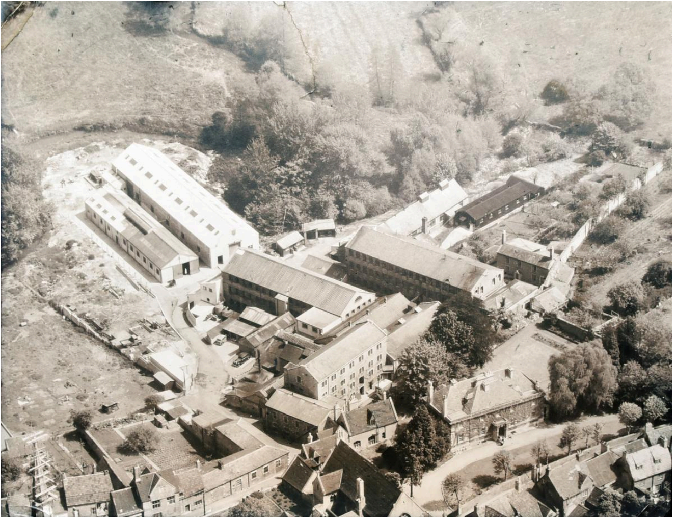
Aerial view of Notts Industries in Saxonvale c1950s
